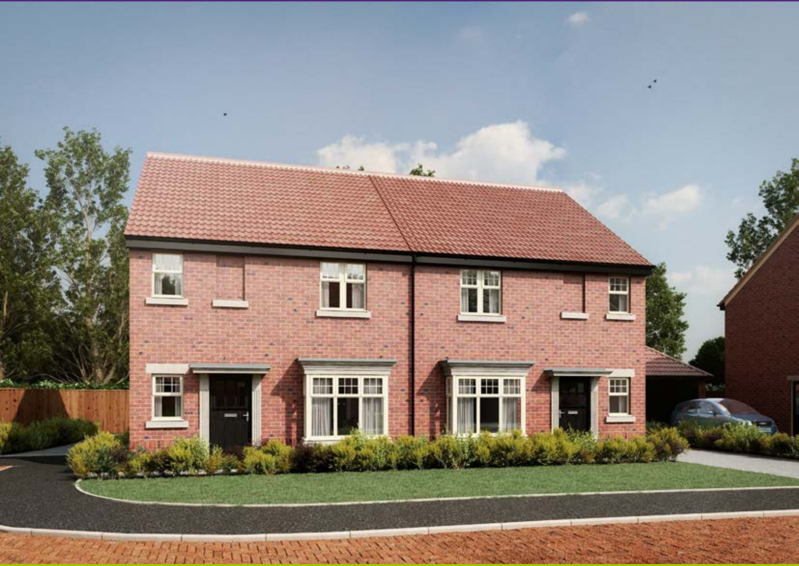
The Curlew (Plot 5), Pavilion Gardens, North Cave, East Yorks., HU15 2NW
