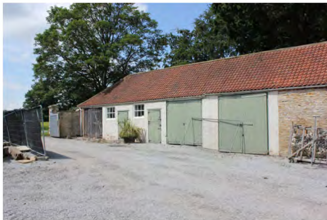
Single storey north range
