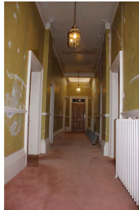
First floor bedroom corridor
