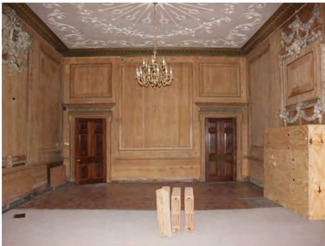
Ballroom, looking north
