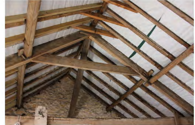
Collared truss with pegged purlin
