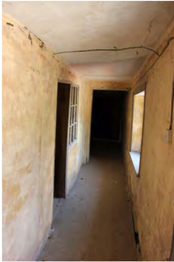
Corridor: note historic plastered walls, lath and plaster ceiling and lime ash or gypsum plaster floor
