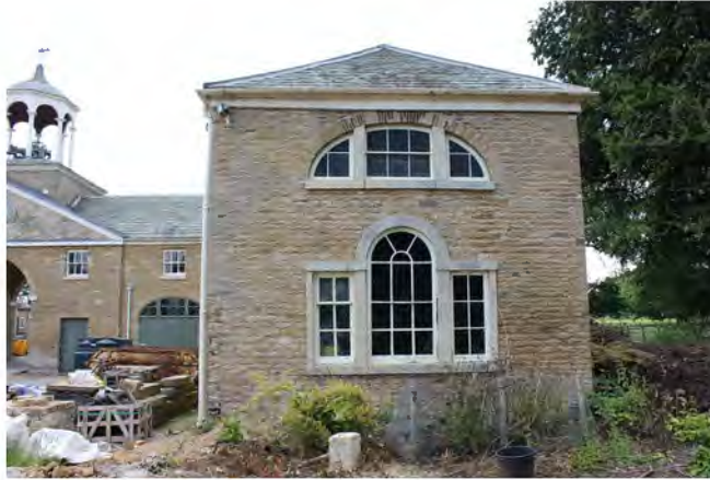
North wing gable end
