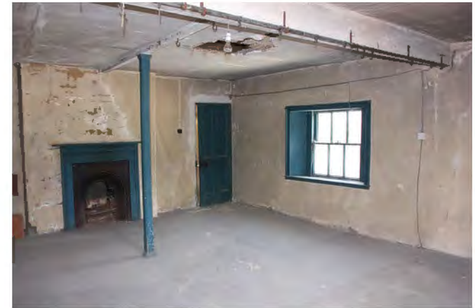
Room above former laundry
