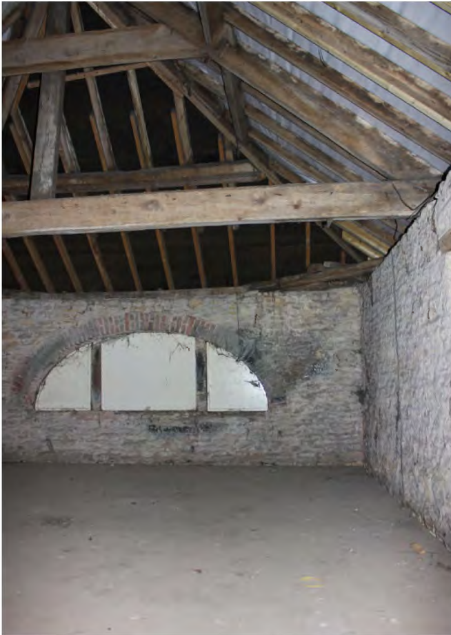
Hay loft or feed store with blocked Diocletian window with brick arch and stone mullions
