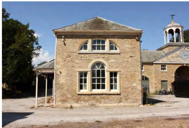
South wing gable end
