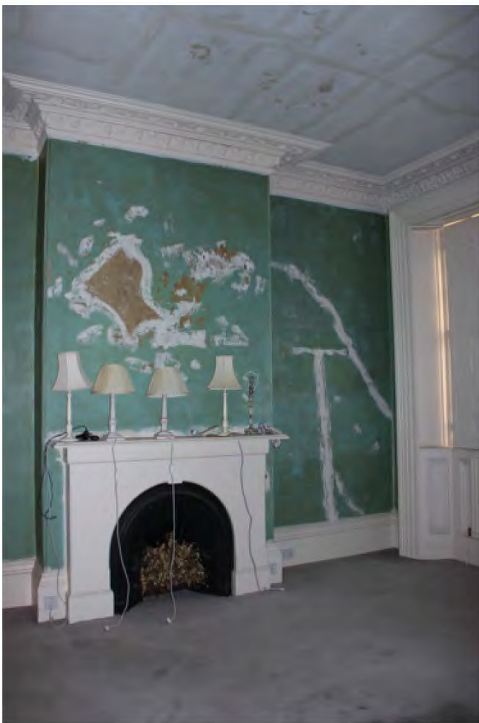
Bedroom FF12 with decorative cornice, marble fireplace and cast-iron grate and window shutters
