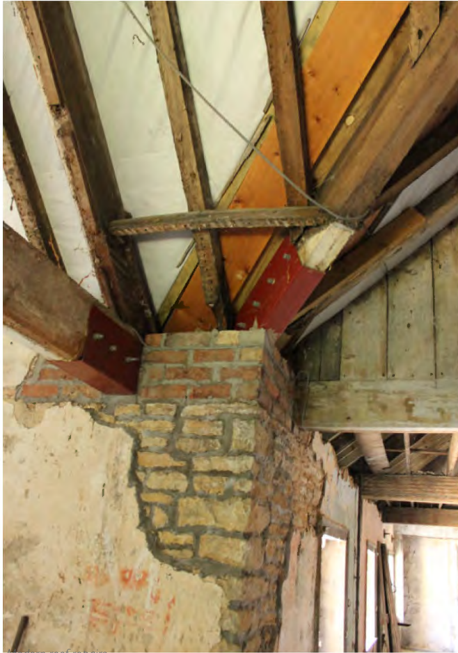
Modern roof repairs
