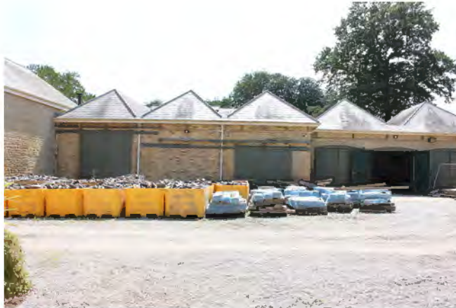
South courtyard range
