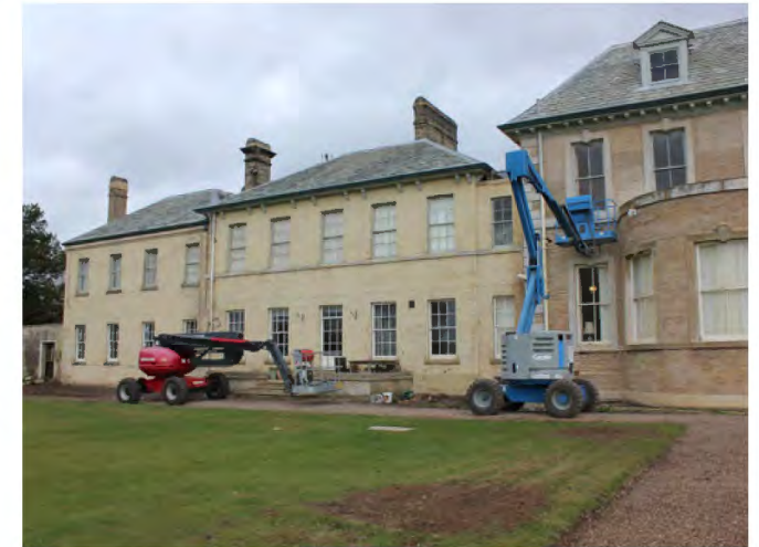
South elevation, west wing
