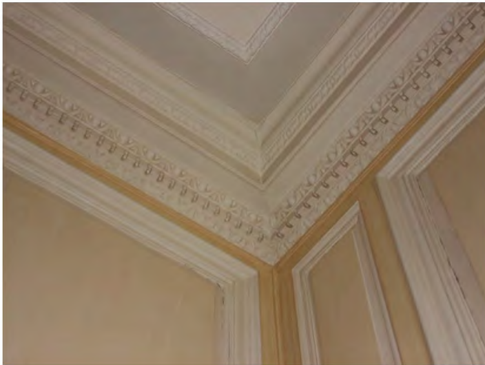
Heavily moulded cornice in the Drawing Room.
