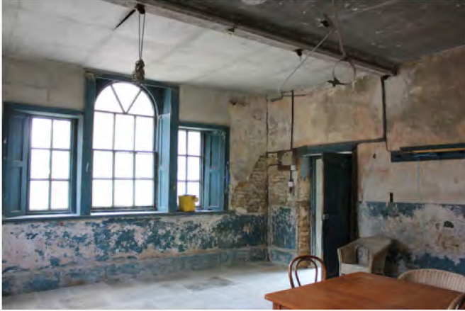
Venetian windows to possible former laundry
