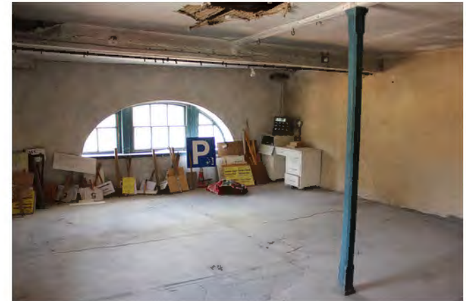
Room above former laundry
