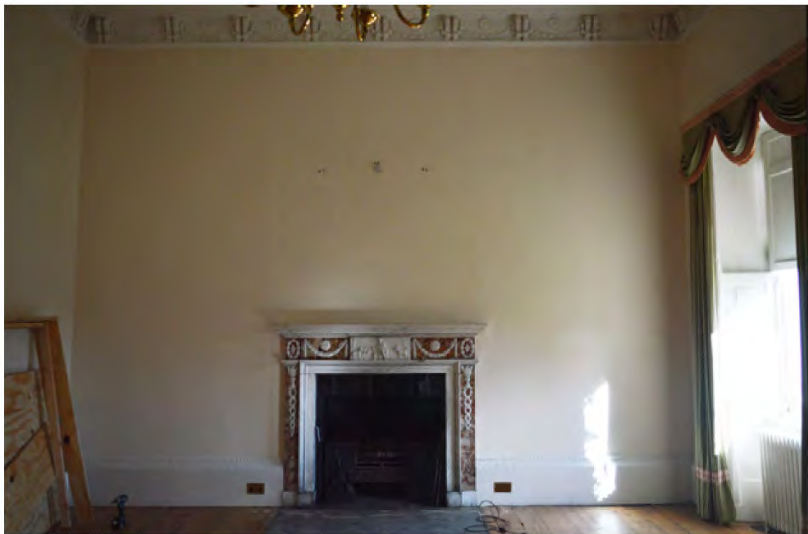
Library, looking east
