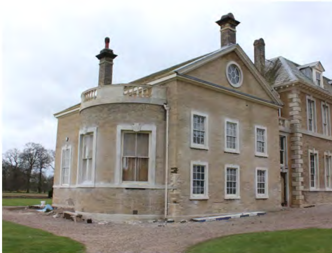
Pavilion northern elevation and bay window
