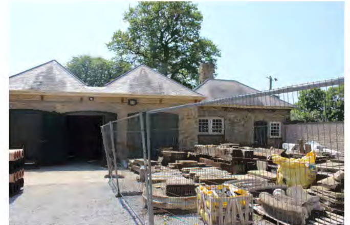
Westernmost building to courtyard
