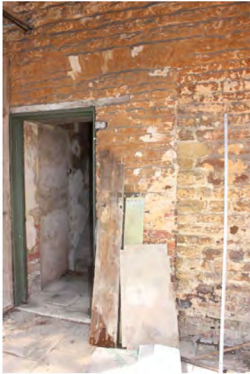
Door to staircase in south wing – note the former opening, now blocked to its right.
