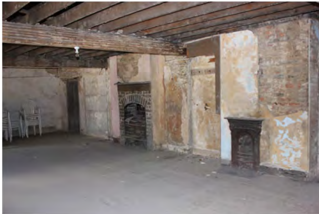
North wall with fireplace and range
