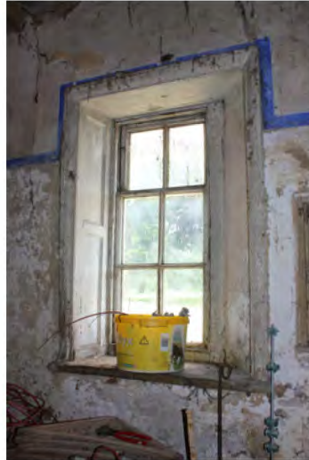
Stable window with bolection moulded architrave
