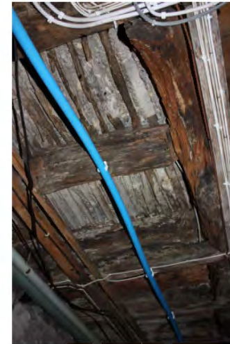
The underside of laths in the cellar plastered from above, providing evidence of a possible lime ash or gypsum plaster floor on the ground floor former service corridor in phase one
