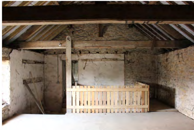
Stair with plastered walls to former enclosure
