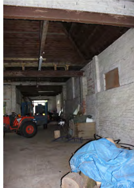
Central range looking east
