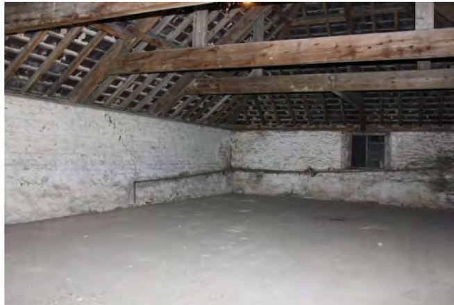
Loft above western extension, looking north
