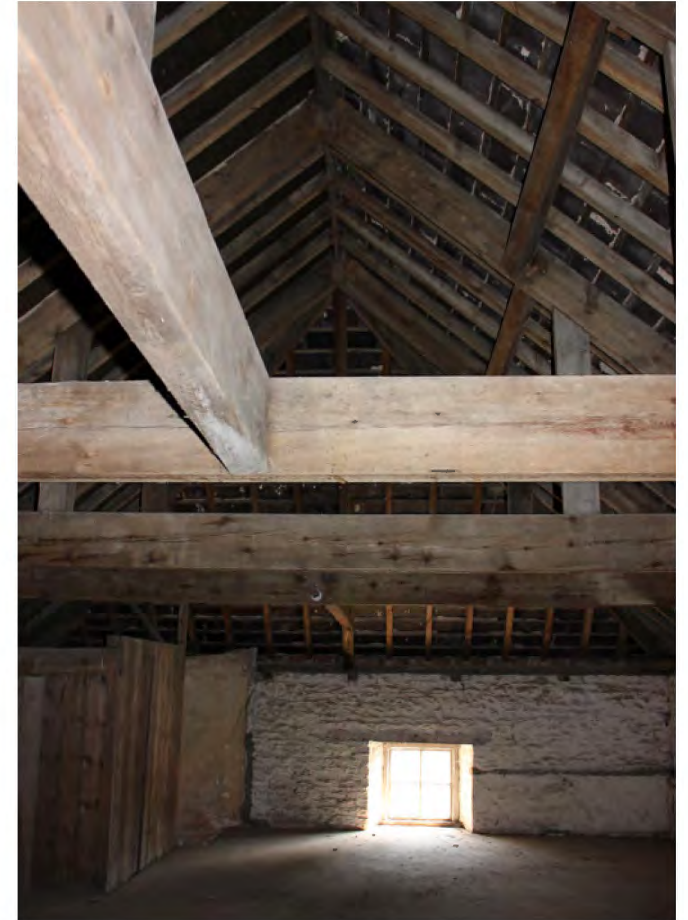
Loft above western extension, looking south
