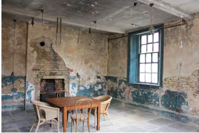
Possible former laundry
