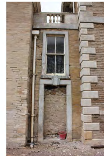
Blocked door with lowered window above to pavilion link
