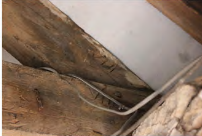
Carpenters marks to aid assembly
