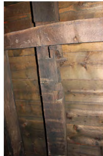
Evidence of reused timbers
