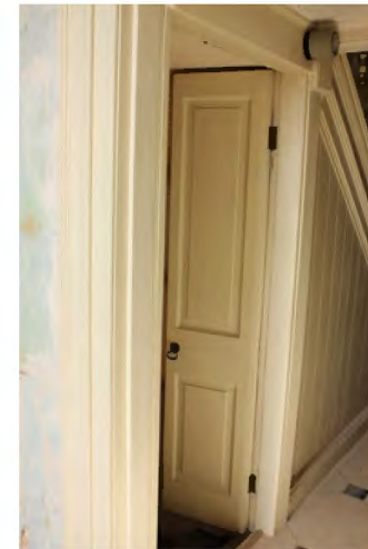
Phase 1 entrance to cellar - note the doors are later
